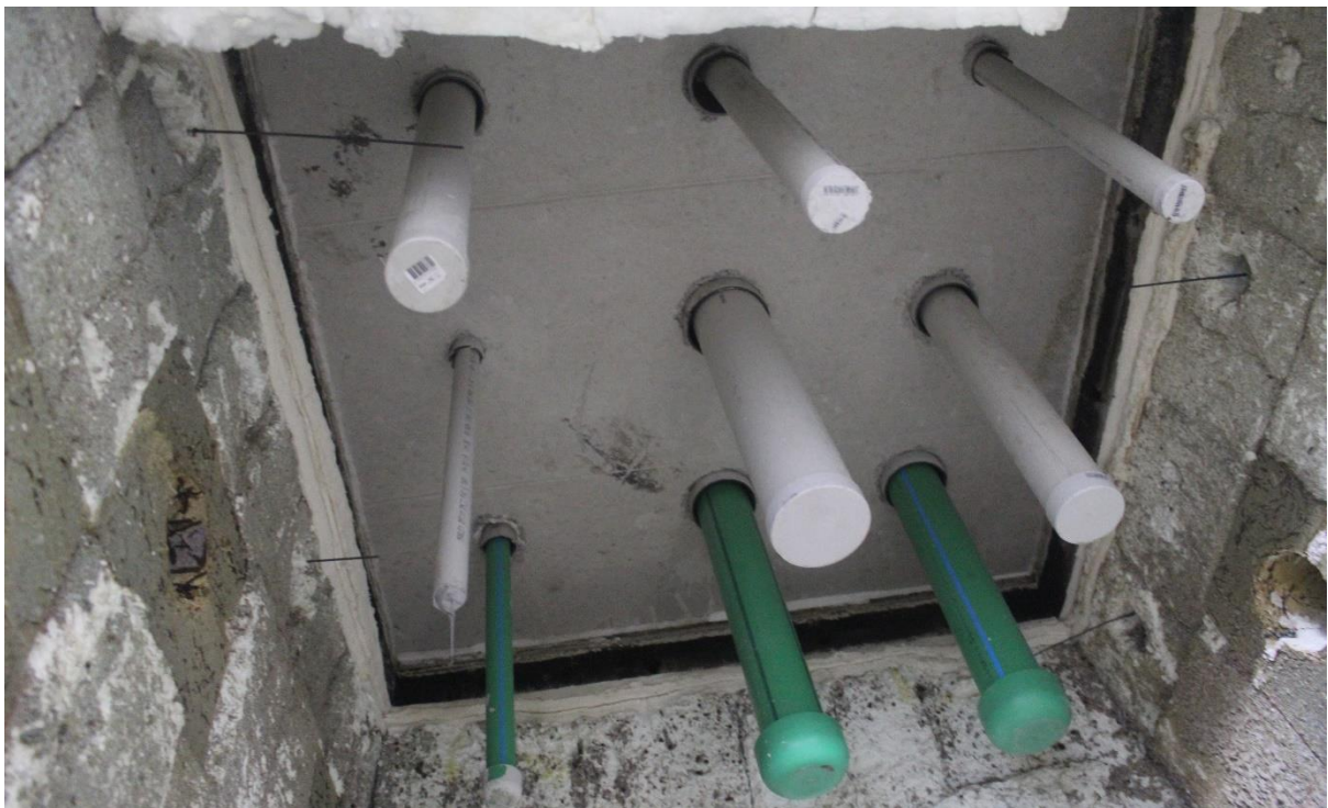
Figure 22 – Exposed face prior to test commencement
